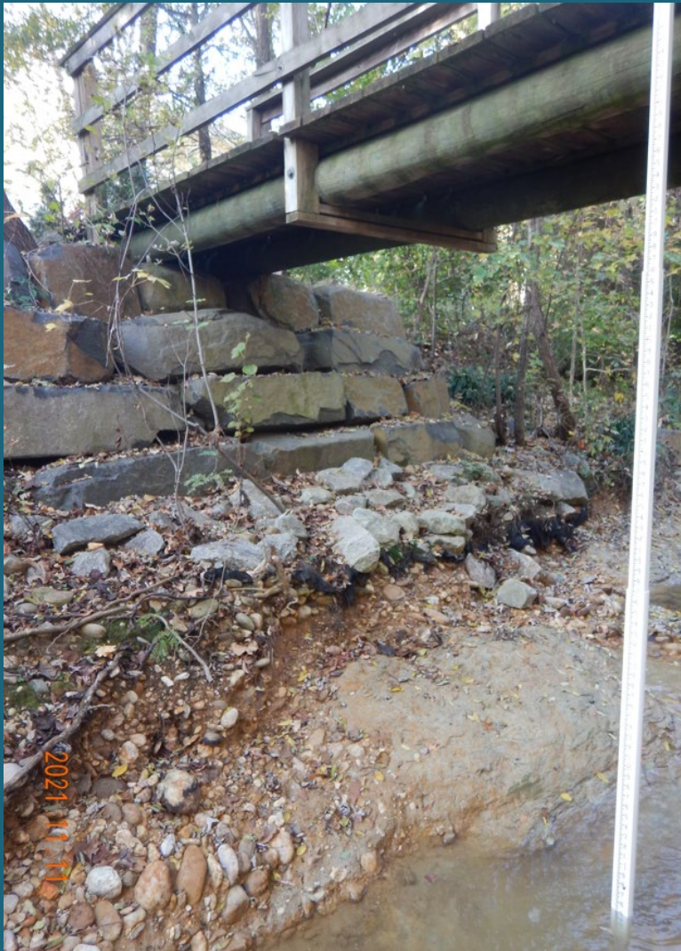
November 2021; Underneath Bridge
