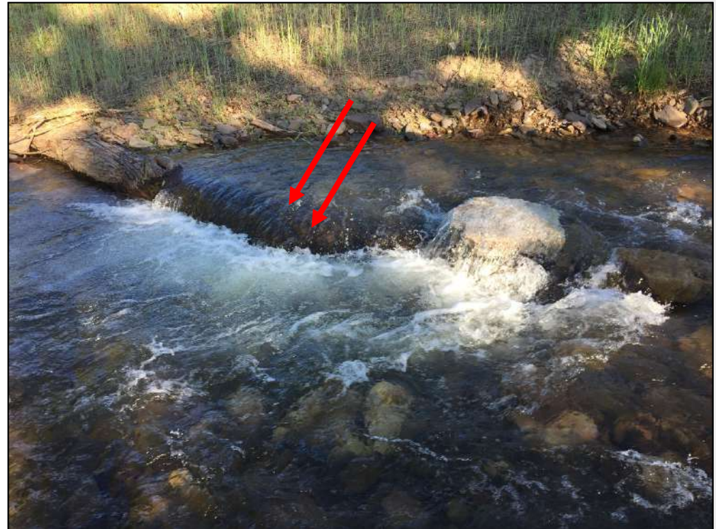
Log Vane Structure
