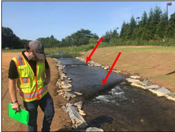
Cascade with Log Rollers
