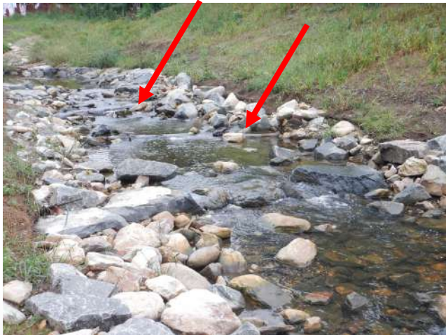
Cascade with Log Rollers
