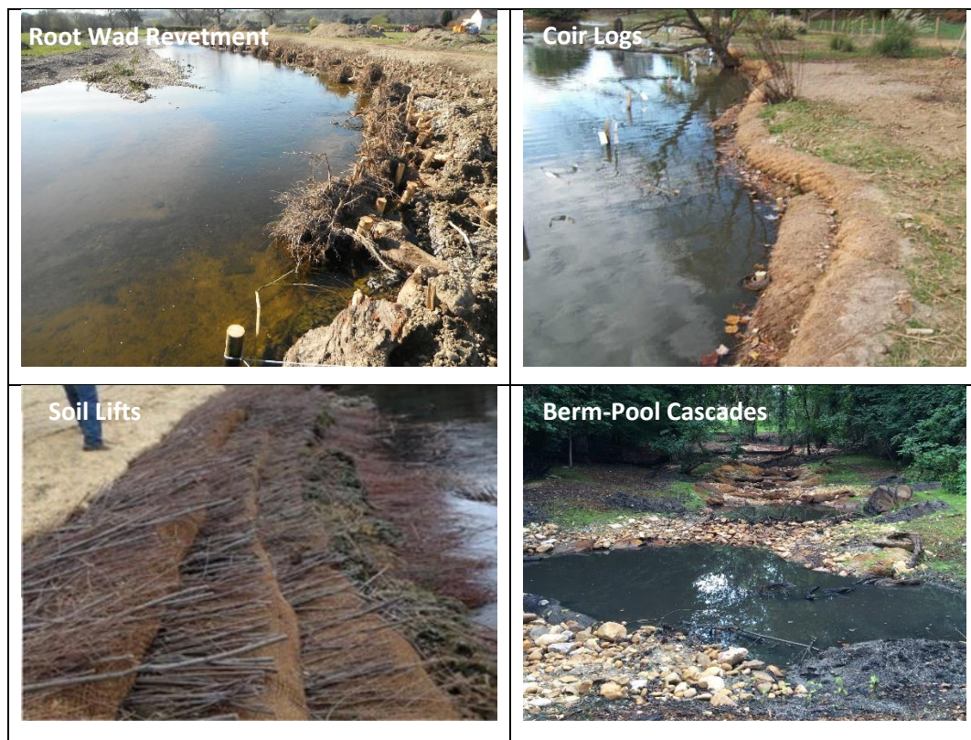
Figure 6. Examples of “credible” armoring practices.
