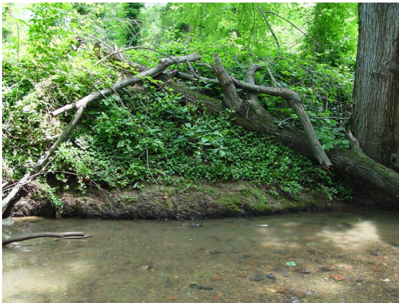
Figure 14. Suspended log bank protection.
