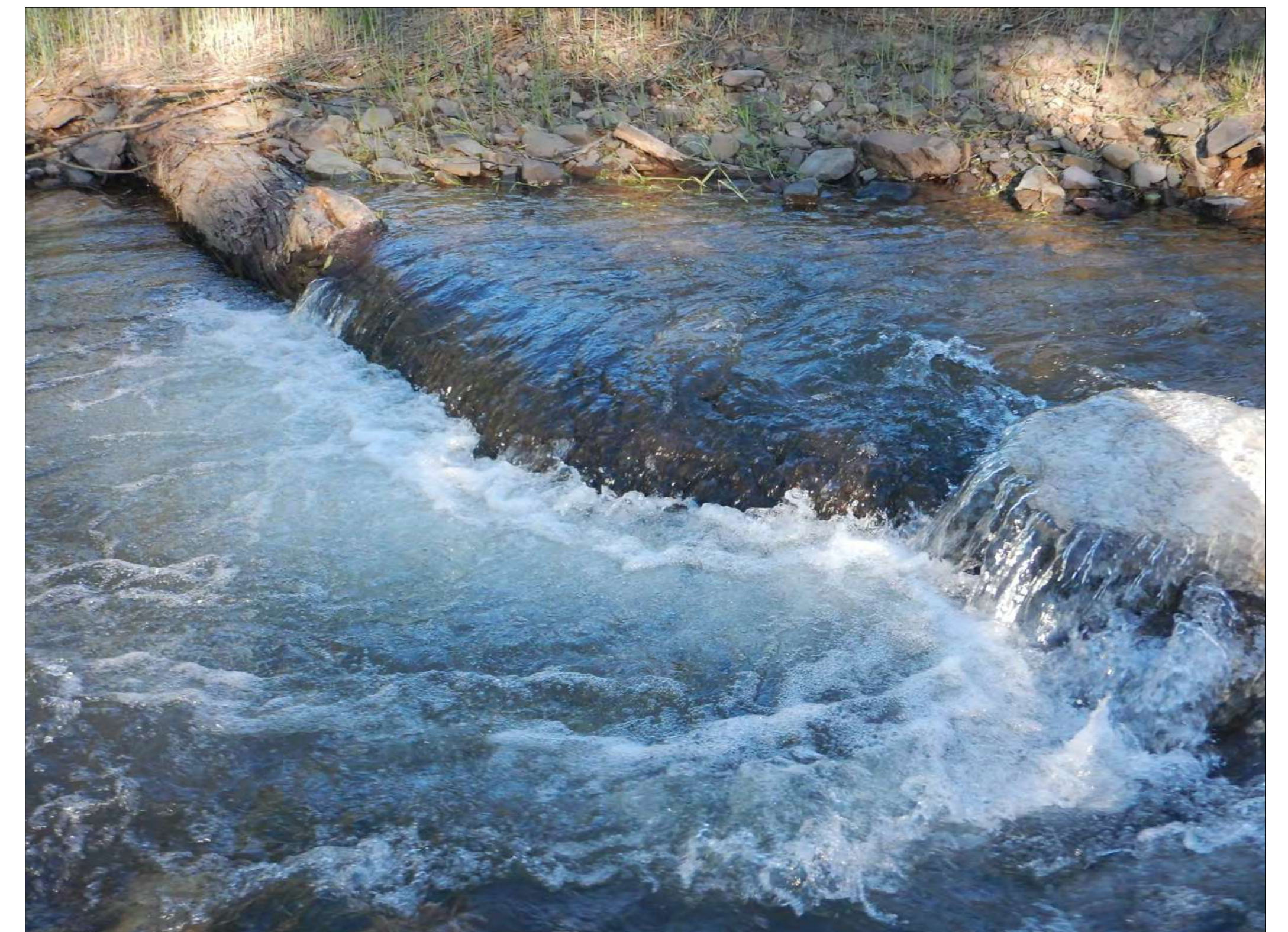
EXAMPLE CONSTRUCTED LOG VANE
