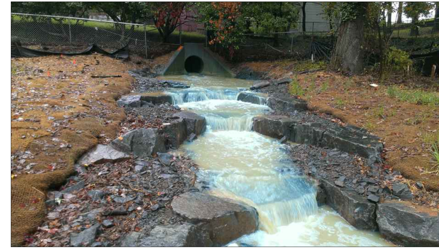
CONSTRUCTED PLUNGE POOL (SHOWN FOR INFORMATION ONLY)
