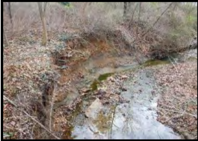
FIGURE 2: Abandoned meander sitting about 3-feet higher than the existing stream bed
