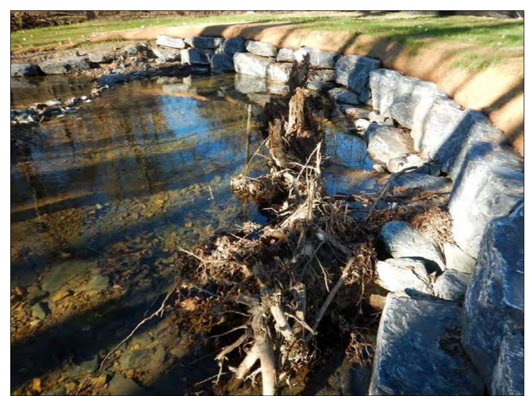
EXAMPLE ROCK WALL WITH TOE WOOD
