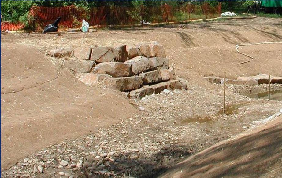
Left bank looking upstream
