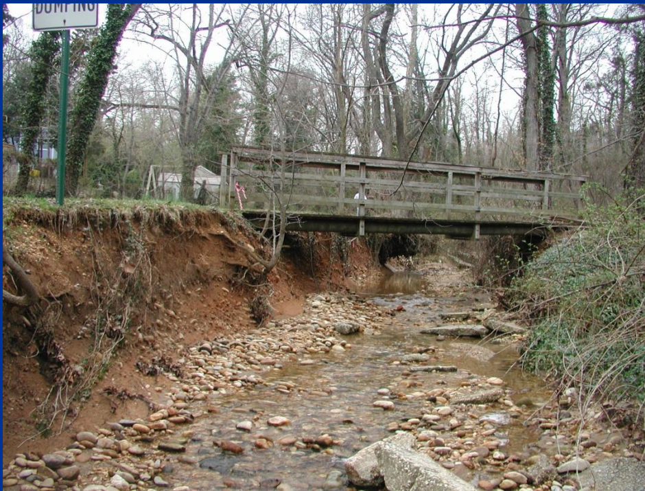
Looking upstream toward bridge (2005)
